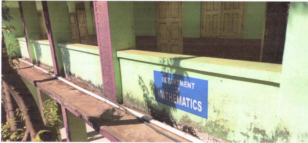
Photograph of Rain Water harvesting pipe
